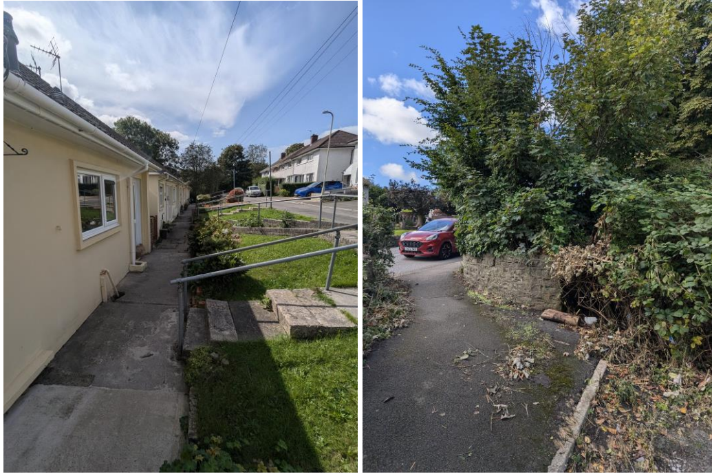
Figure 26 & 27 – Hafan Y Bryn Properties & Culvert Inlet Post Vegetation Clearance
