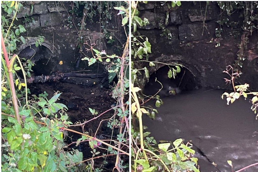
Figures 24 & 25 Network Rail Culvert downstream
